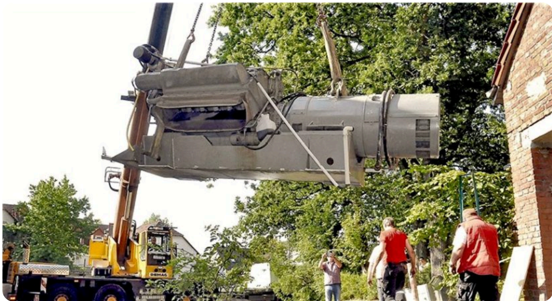
Abb. 4: Notstromaggregat
